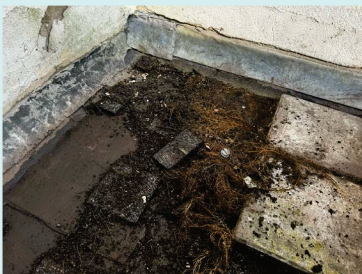
Survey/inspection of roof due to leakage
